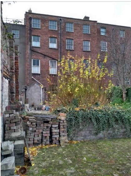
4 Henrietta Street rear elevation. View from inside former mews.
