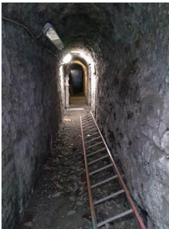
View of underground tunnel and vaults located underneath garden of 4 Henrietta Street. The door at the northern end of the vaults leads to further vaults which support the upper floor of the former mews building.
