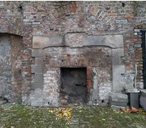
Detail of granite fire surround, flanked by niches, to east gable wall of former mews building.
