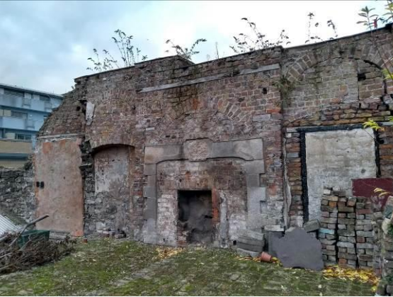
View of surviving east gable wall of former mews building with remains of large granite fire place. This fireplace vented into the large chimney which can be seen in the photo of the original mews building on the right.
