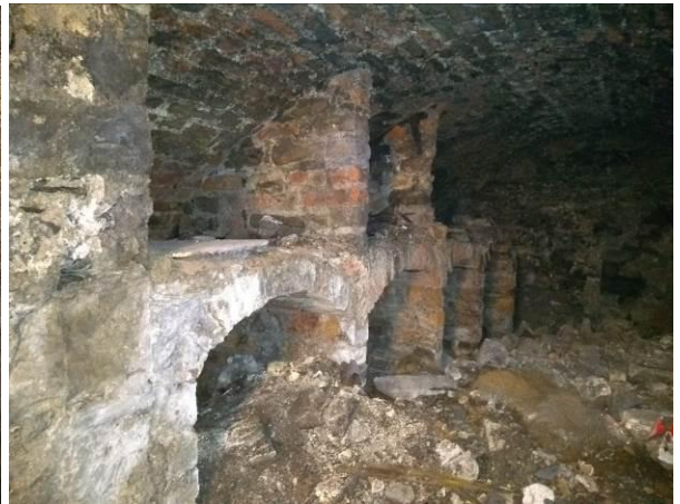
View of underground tunnel and vaults located underneath garden of 4 Henrietta Street. The door at the northern end of the vaults leads to further vaults which support the upper floor of the former mews building.
